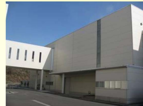
Constructed in the No.3 Production Building at the Takahagi Plant
