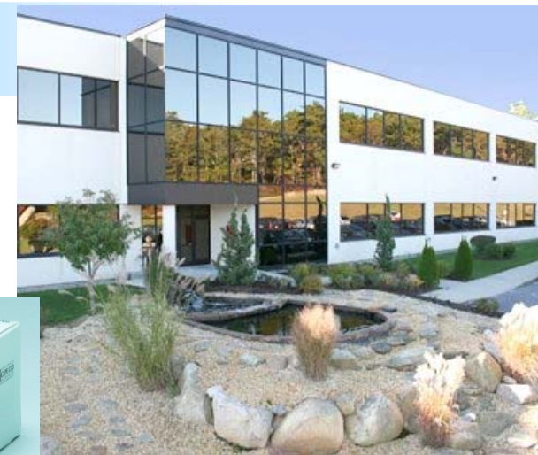
Exterior of the ACC offices
