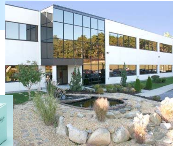
Exterior of the ACC offices
