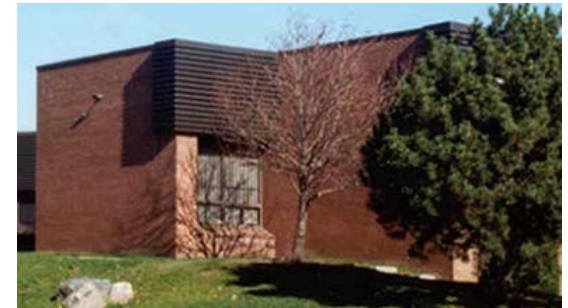
Exterior of the Dalton offices
