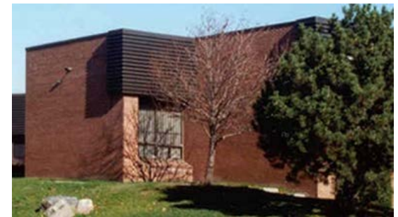
Exterior of the Dalton offices
