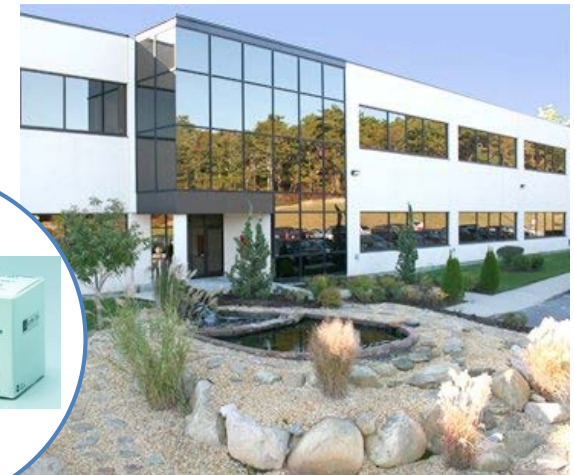
Exterior of the ACC offices
