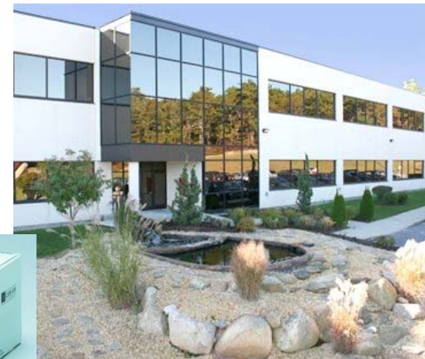
Exterior of the ACC offices
