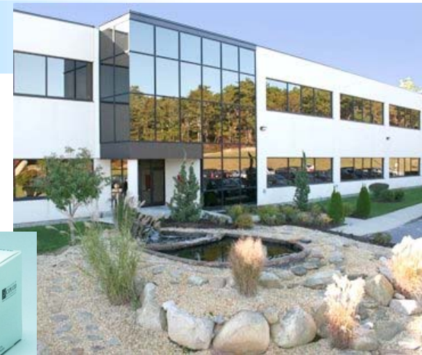
Exterior of the ACC offices
