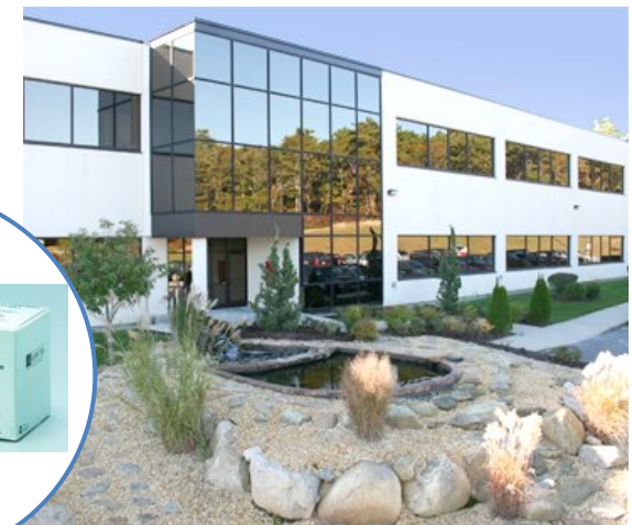
Exterior of the ACC offices
