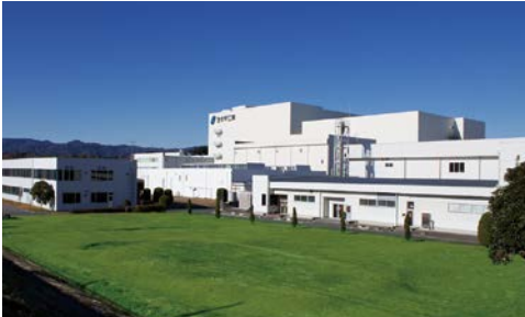
Seikagaku Corporation Takahagi Plant (Ibaraki Prefecture, Japan)
