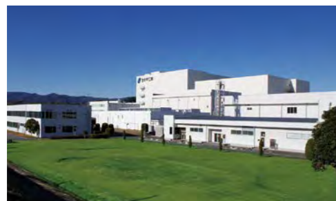
Seikagaku Corporation Takahagi Plant (Ibaraki Prefecture, Japan)
