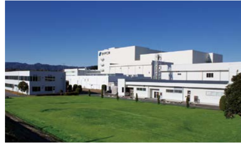
Seikagaku Corporation Takahagi Plant (Ibaraki Prefecture, Japan)
